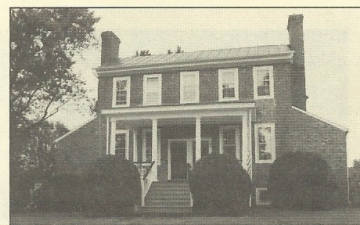
Cool Water, now the home of Virginia delegate Frank Hargrove, was built in 1735
